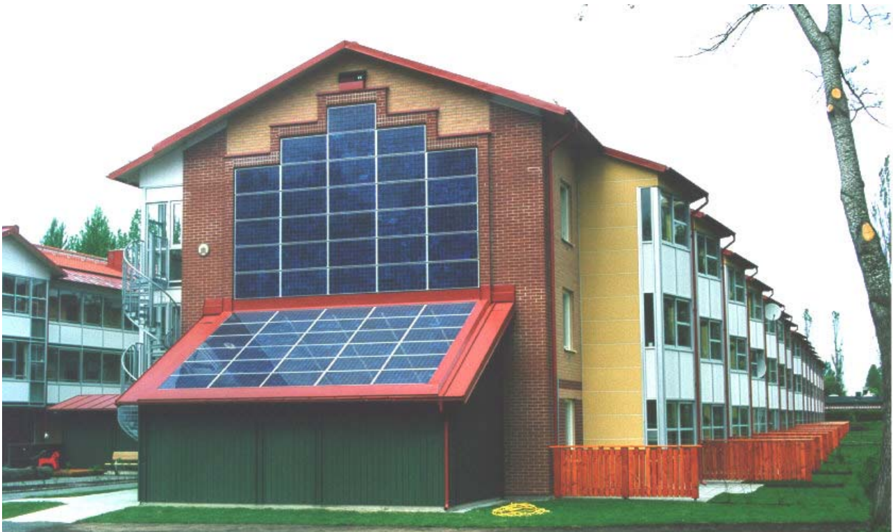
Solar modules were mounted on a residential apartment's building gable in a renovation project.
