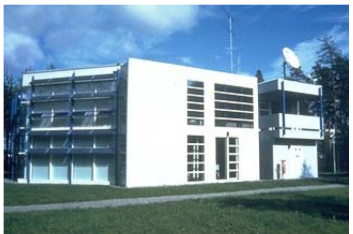
Low energy private house uses solar modules which are integrated into shading devices.
