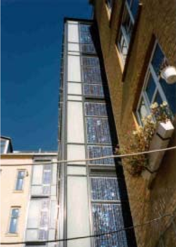
In this building in Copenhagen the solar modules have been fully integrated into the facade and they are directly connected to ventilation fans.
