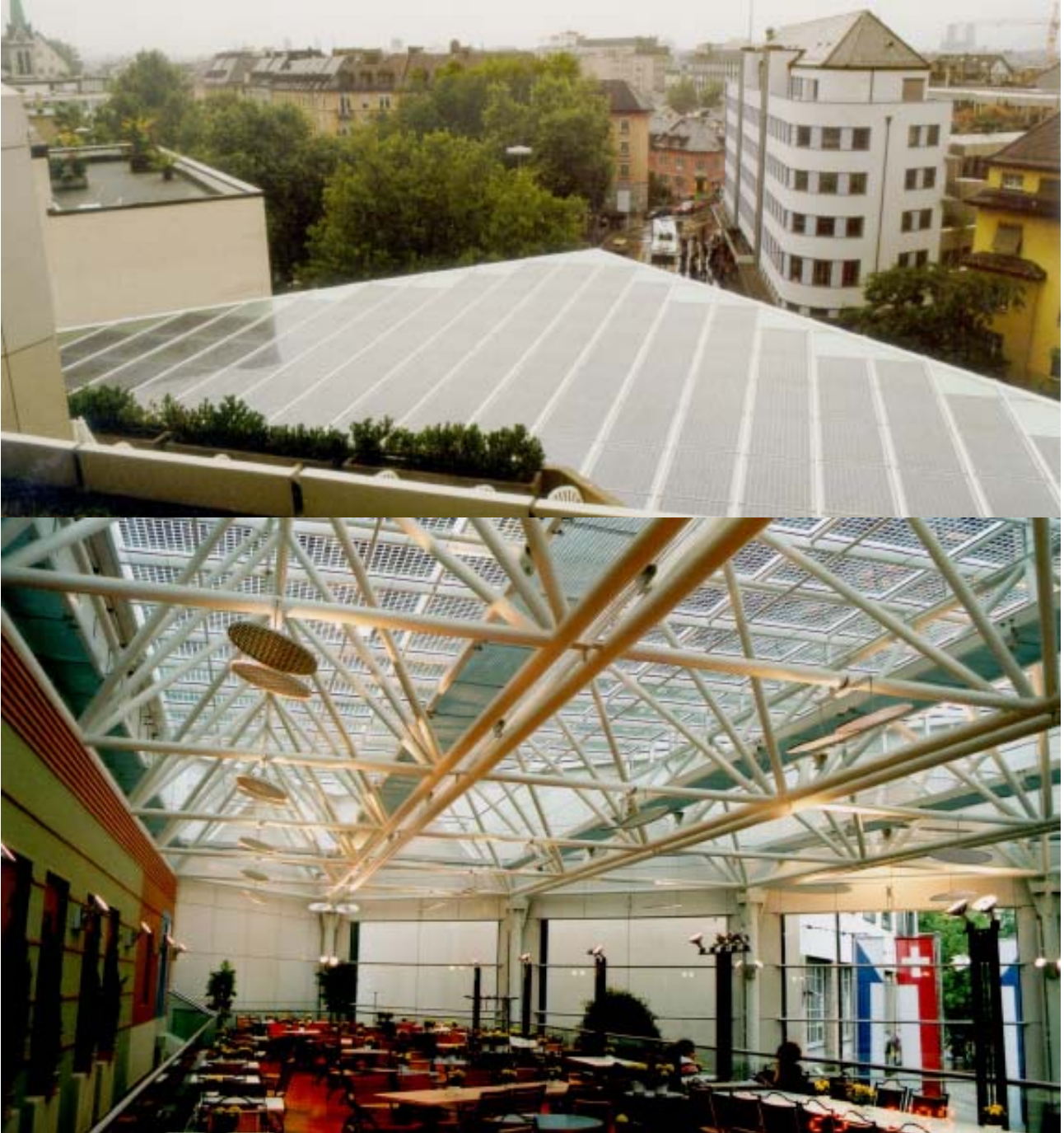
Commercial building roof-tops and façades provide an ideal mounting for large areas of solar modules, which can act both as electricity generators and as decorative elements. Outside and inside view of an entrance hall's glass roof that also serves as a sun protection glass reducing overheating.
